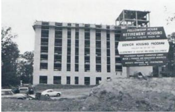
Lake Anne Fellowship House under construction in 1970
