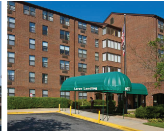
Largo Landing Fellowship House (1984) is home to 105 residents.
