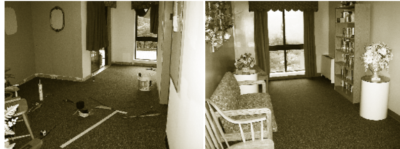
Lake Ridge's common area carpets are being replaced and new floor expansion joints inserted.
