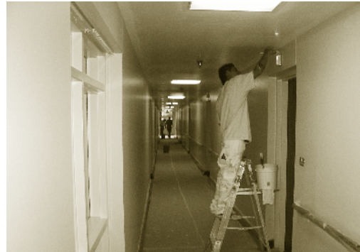
New paint refreshes Largo Landing's hallways.
